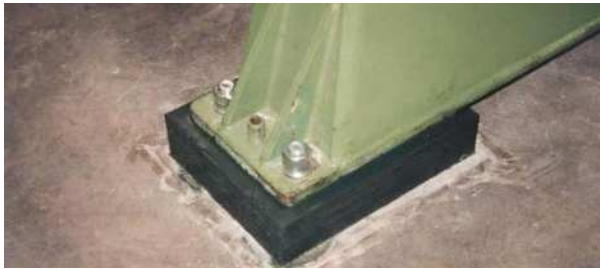
Figure 7. Machinery Mounted Using an Epoxy Resin.
