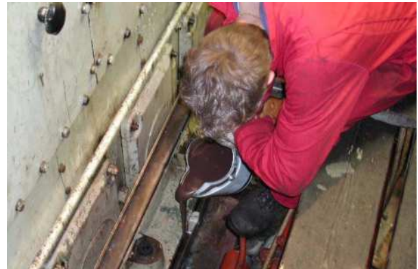
Figure 5. Pouring Epoxy Resin.
