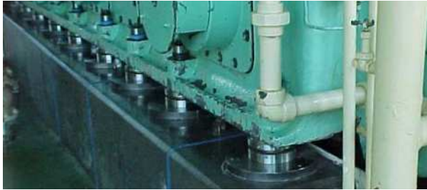
Figure 3. Vibracon® SM Element Application on Concrete.
