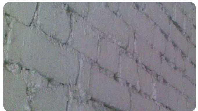
Fig. 2 Dust is captured in open grouting.
