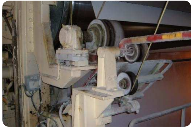
Fig. 7 Dust collects on shafts and hubs.
