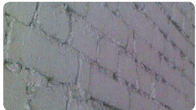
Fig. 2 Dust is captured in open grouting.
