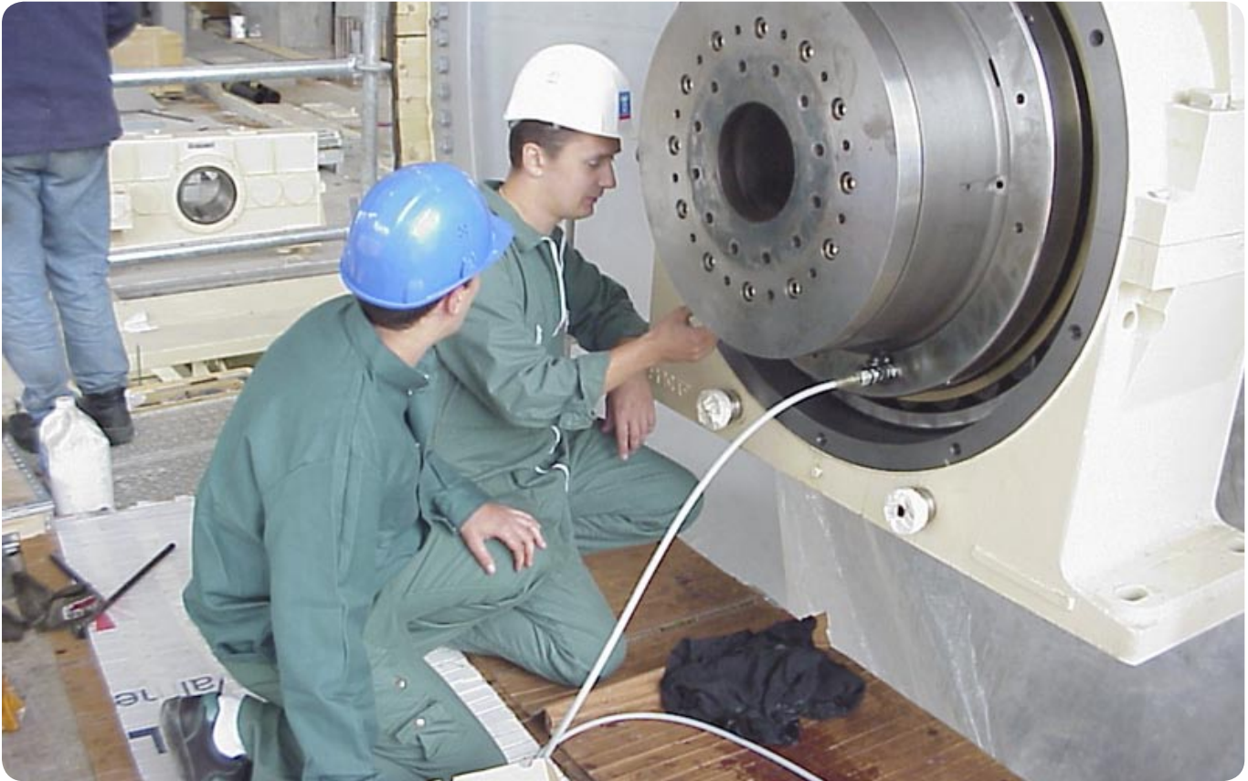
Mounting CARB toroidal roller bearing on a Yankee cylinder using the SKF Drive-up method
