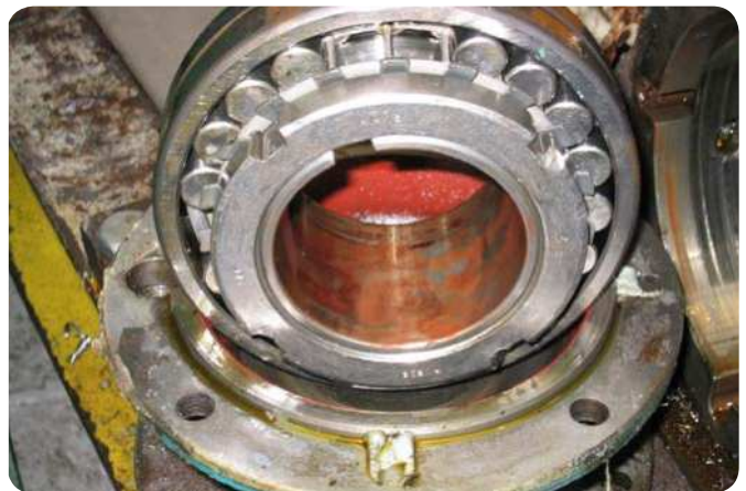
Fig. 11 Fretting corrosion in the bore of an adapter sleeve of a dryer section felt roll bearing due to an insufficiently tight fit relative to the load.
