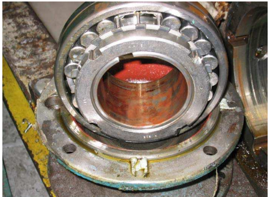
Fig. 12 Heavy fretting corrosion in an adapter sleeve bore, but the bearing raceway is in quite good condition which gives a clue about the root cause
