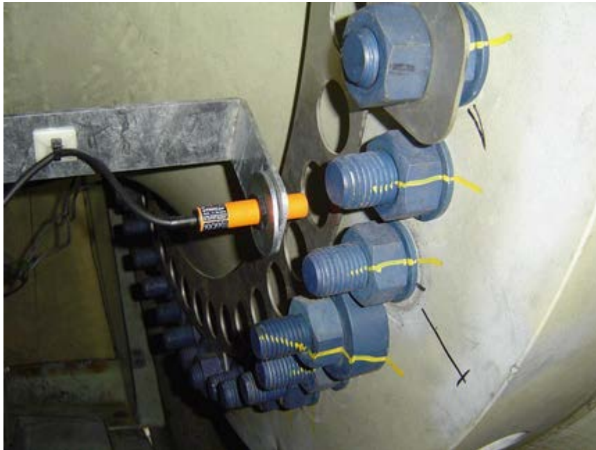
Figure 3 - 18. Connection of Pulse Transmitter.
