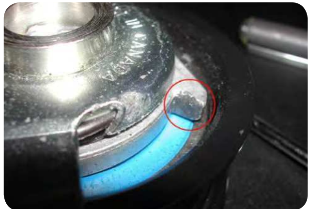
Back plate of tensioner broken, indicator has come into contact with end stop.
