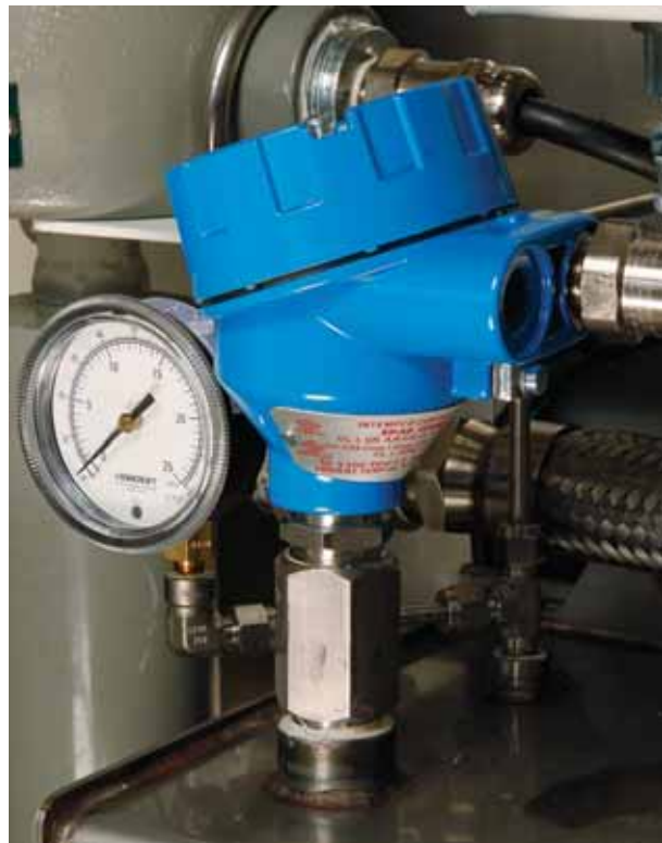
Fig. 12 Mist Pressure Gauge and Oil Level Sensor
