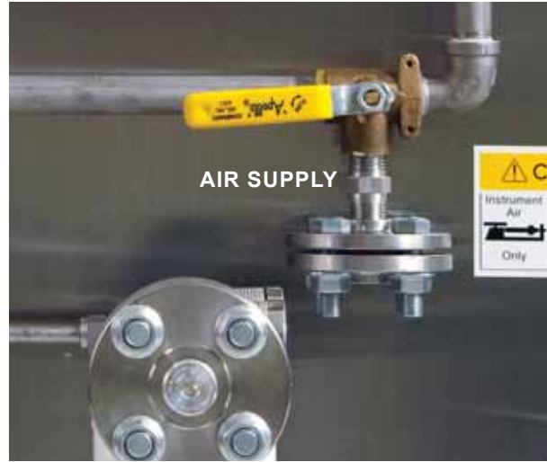
Fig. 08 Air Supply Connection
