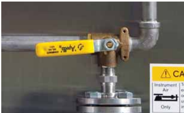
Fig. 22 Air Diverter Valve (Left Side of Enclosure)
