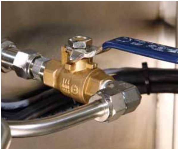
Fig. 18 Oil Refill Shut Off Valve (Inside of Enclosure)
