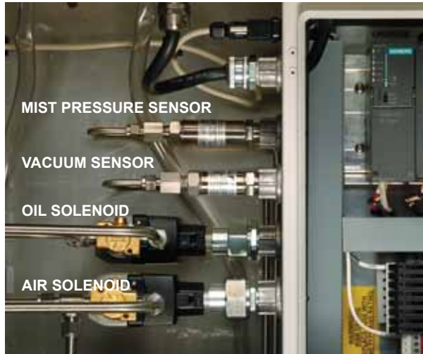
Fig. 10 Air and Oil Refill Solenoids, Pressure and Vacuum Sensors
