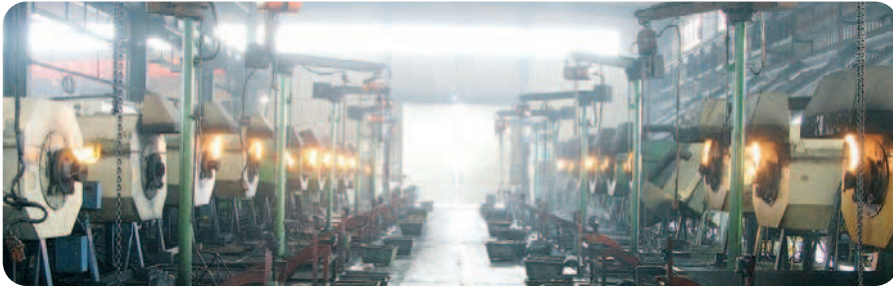
Rotary furnaces used in the heat treatment process provide a uniform heat for a more consistent and uniform result
