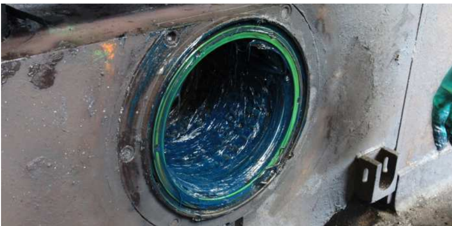
Outer ring and rollers assembly mounted and filled with grease
