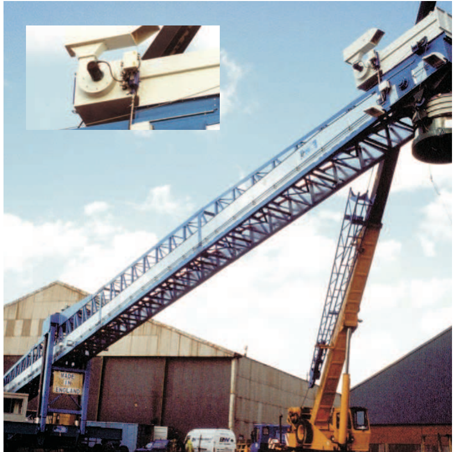
SKF Cooper flange on a ship loading conveyor
